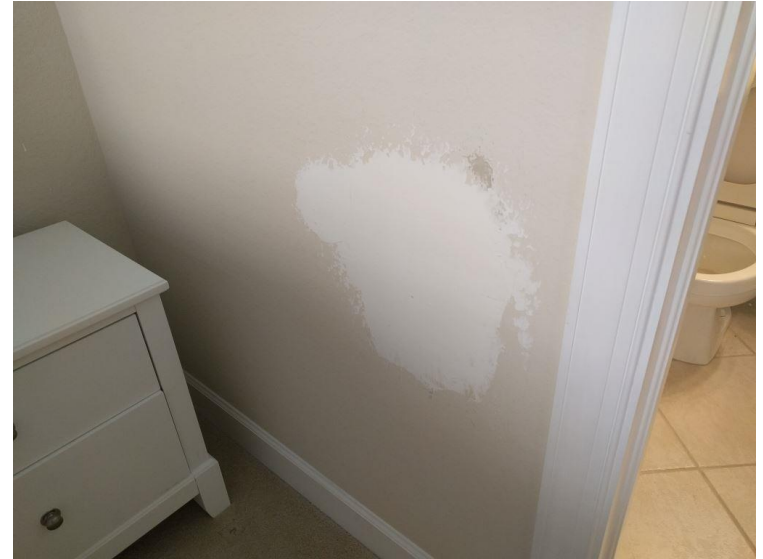
After patching before painting
