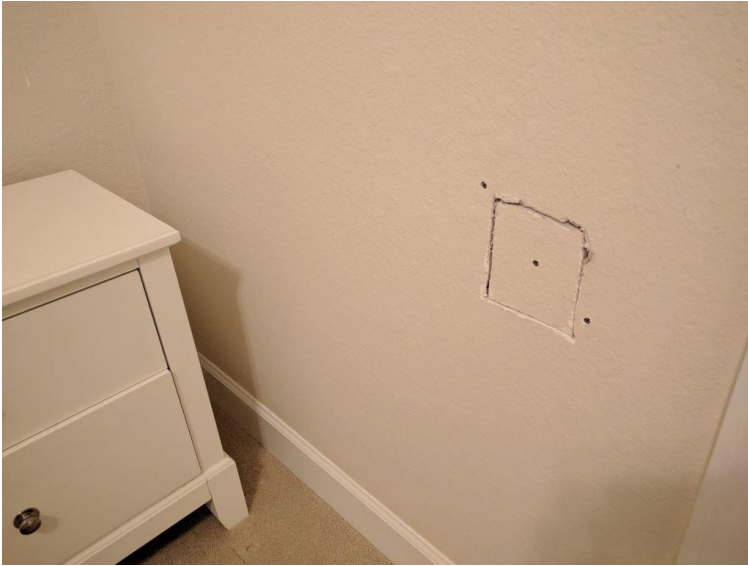
After cutting access to allow wiring to be pulled
