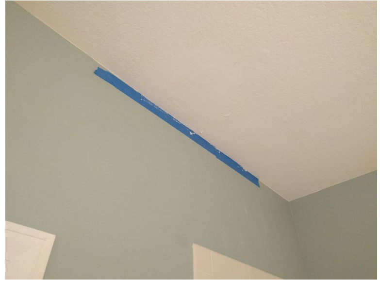
After patching before painting
